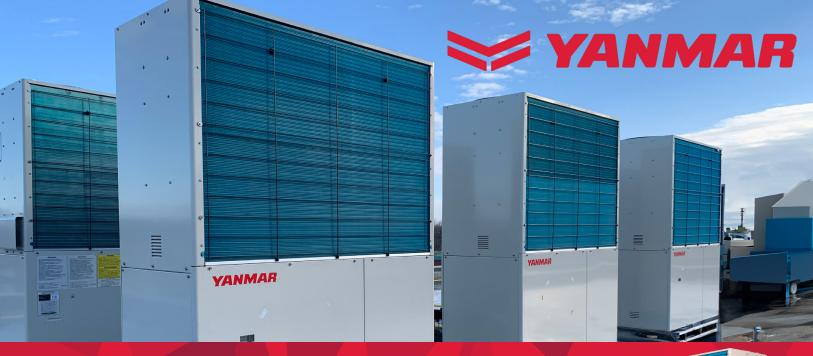
The natural gas heat pumps provided an electrical load reduction of approximately 30% and an 80% carbon emission reduction as compared to electric heat pumps powered by the grid.
